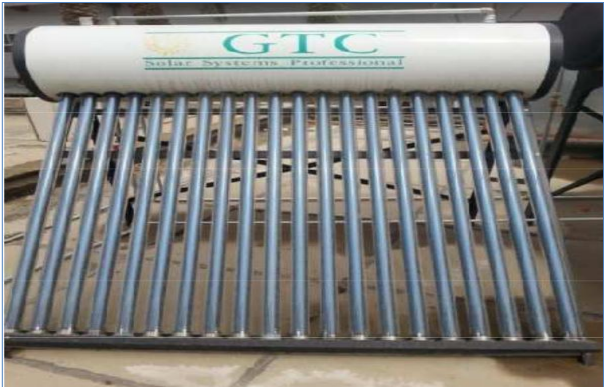
Figure 1: Evacuated tube solar thermal collector [6]
