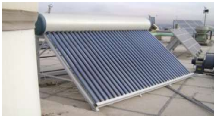
Figure (4): The evacuated tube type solar water heater absorber (ETA) with Tank.
